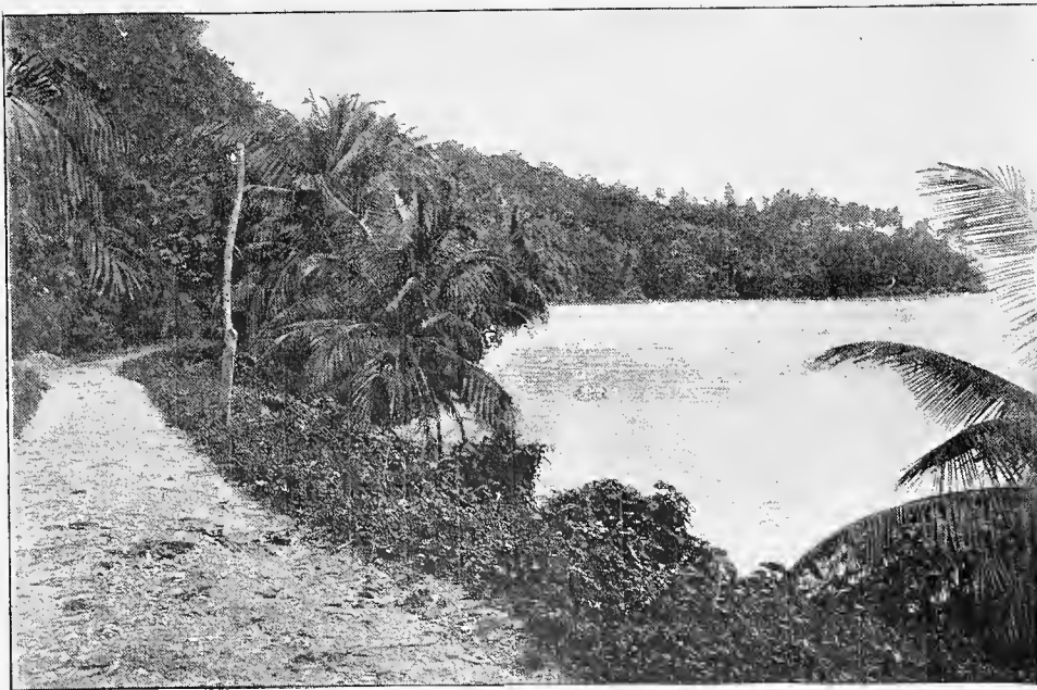
ON THE NORTH COAST ROAD.
